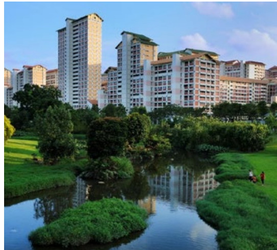
The naturalising of a concrete canal in Bishan-Ang Mo Kio Park through the Active, Beautiful and Clean (ABC) Waters programme.
