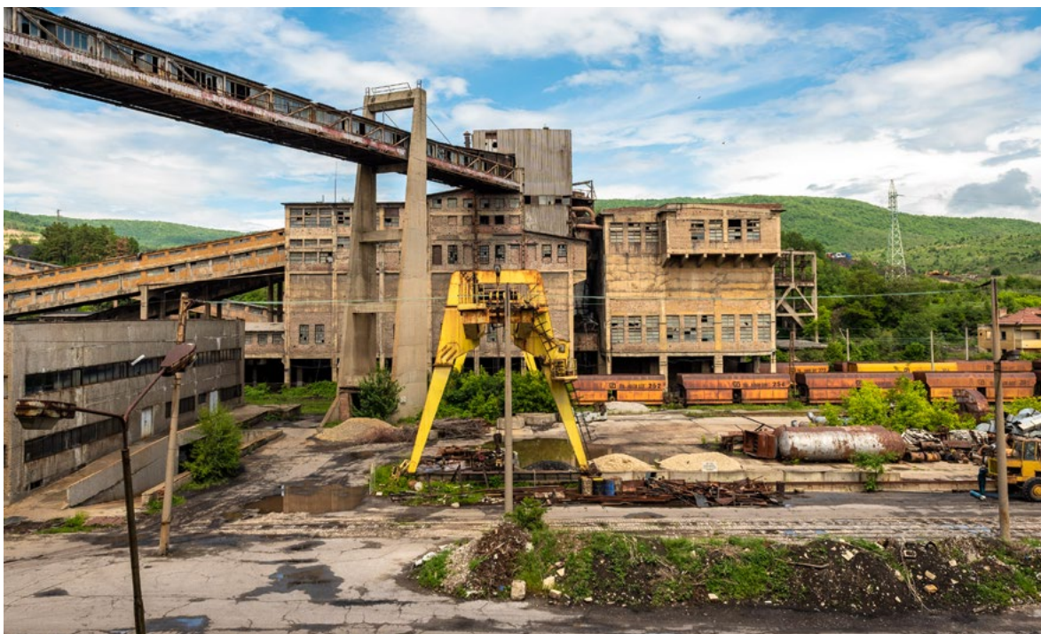
The enrichment factory is still operating albeit at low capacity. It was built around 1944 next to the underground mine Babino which closed at the end of 2016.
