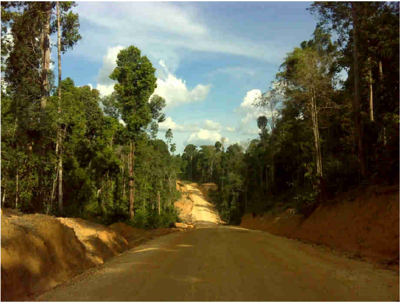
APP logging road through logger-over but still dense natural forest in PT. Lestari Asri Jaya concession, block #13 © WWF-Indonesia, 1 June 2010 at S1°12'34.78"; E102°29'59.83".
