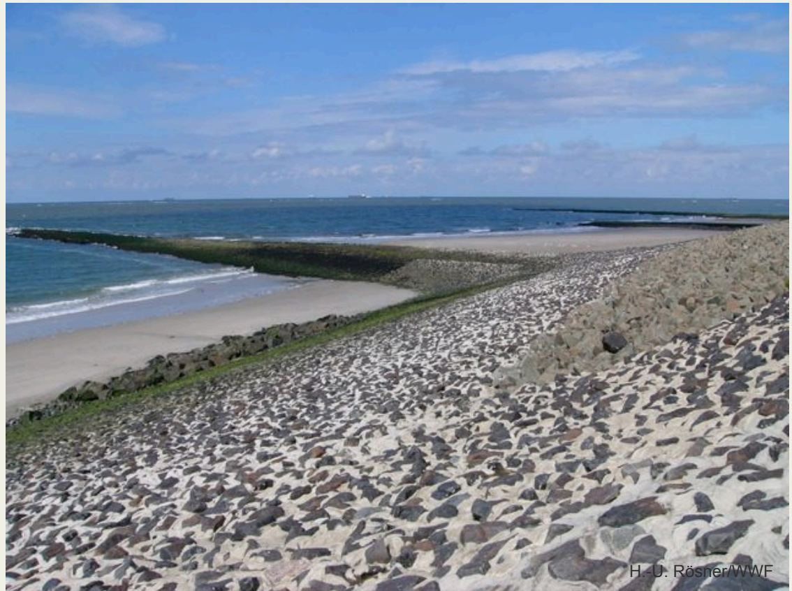
Dike made of rock on the island of Wangerooge
