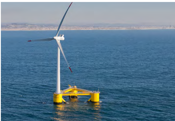
A prototype floating wind turbine, approximately 5km offshore of Póvoa de Varzim, Portugal
