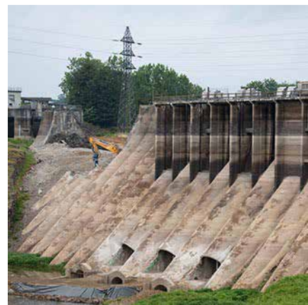
Le Vezin Dam at Selune River, Normandie, France © Roberto Epple
